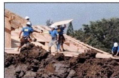
Workers move quickly to build one of two structures going up at the "Extreme Makeover" site. The project is a round-the-clock effort.
