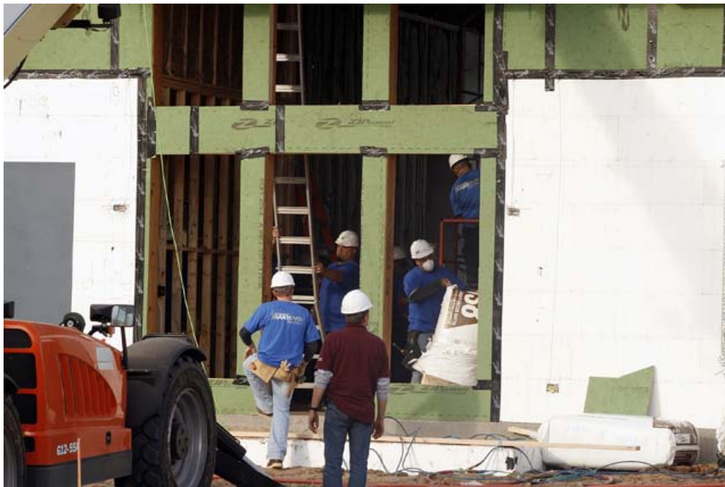
Volunteers were putting insulation into interior walls on Sunday afternoon.
