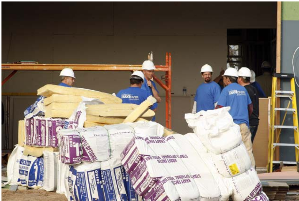
Sheetrock can be seen on the walls of the garage.
